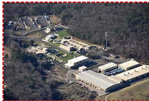
FIG.55 SEWAGE TREATMENT PLANT
