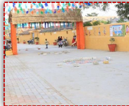
FIG.3 RCC ROAD & PAVING BLOCK
