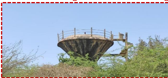
(FIG.34 OVERHEAD WATER TANK)
