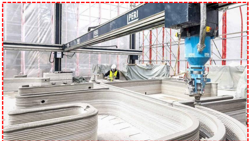
FIG.50 3D PRINTING CONSRTUCTION
